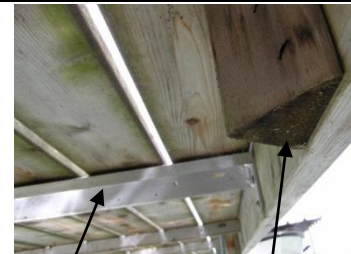
Under Dock Decking Support
