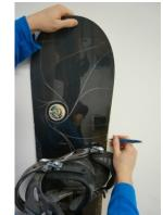
small VERTICAL lines on the wall along the edges of the board, about 2-inches above the upper board binding. Next place one <u>straight HORIZONTAL line</u> on EACH SIDE of your board intersecting with the original Vertical lines. Use a level to Check and ensure 2 horizontal lines are level.
