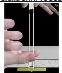
Hold ends of straps between thumb and forefinger and pull toward you until channel rests flush behind decking. Slide plastic cap along straps with other hand until flange of cap is flush with decking.
